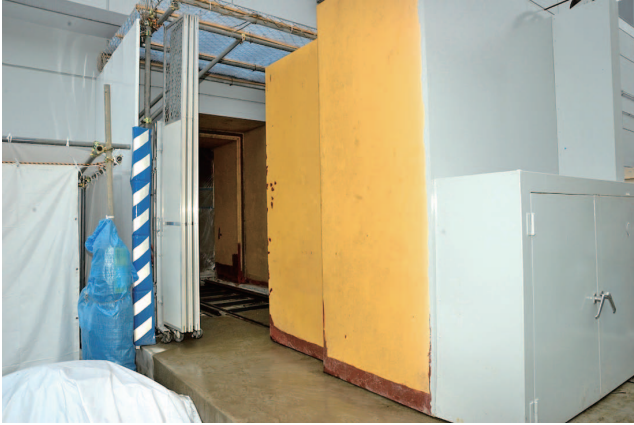
Fig. 10. Repair work on shielding door.
